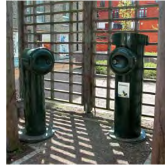
Image 79 Domestic waste chutes to underground storage, Malmö
